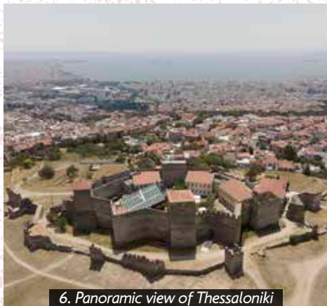
6. Panoramic view of Thessaloniki from Eptapyrgion to the port.
